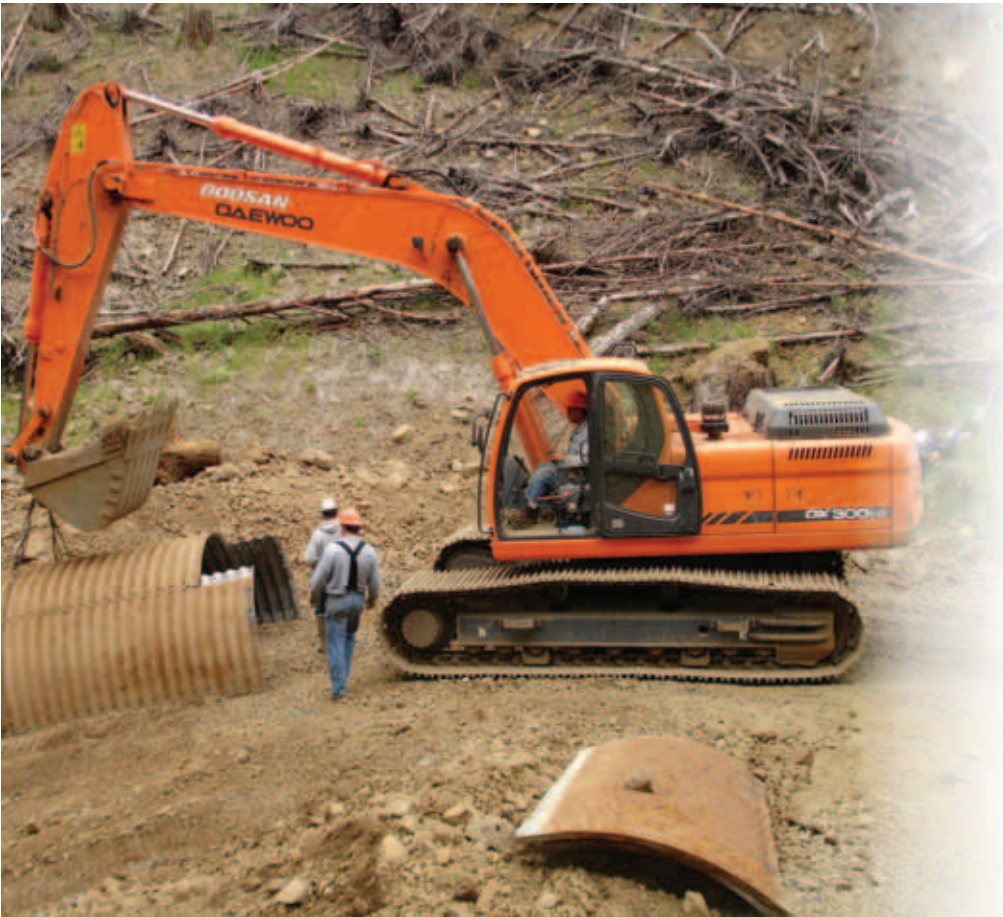
Green jobs in the forest. Workers remove a culvert to improve water quality and salmon habitat on Le Bar Creek in the South Fork Skokomish River watershed in July 2008. Photo by The Wilderness Society
